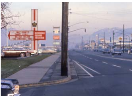
No. 3 Road looking north with sign to Richmond Square Theatres, 1977
