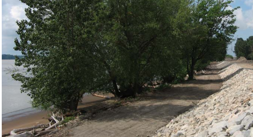
Before and after a dike improvement project which enhanced intertidal habitat and the City's flood protection defences
